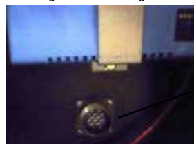
9 ft long Controller wiring harness with male plug located inside ATS
