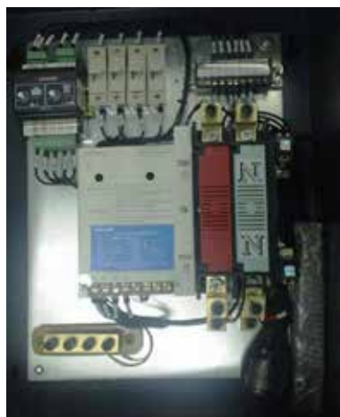
9 ft long Controller wiring harness with male plug located inside ATS
