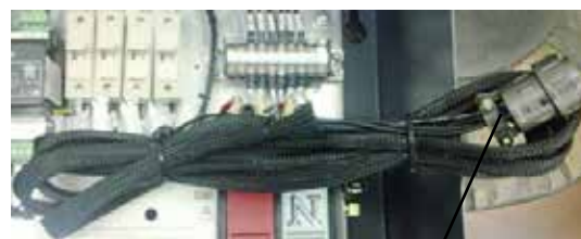
9 ft long Controller wiring harness with male plug located inside ATS
